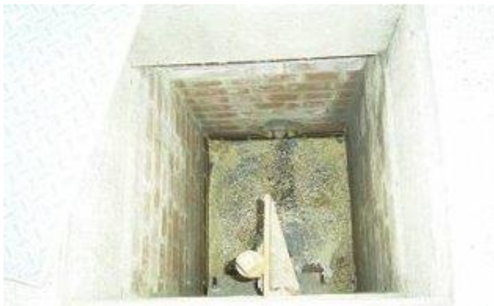
Previous Outfall 1 sampling point
